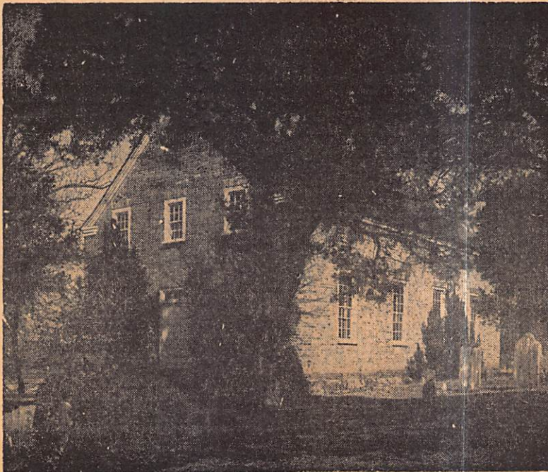
OLD BRICK CHURCH ERECTED 1788
